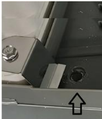
Image: Access to internal drain line
